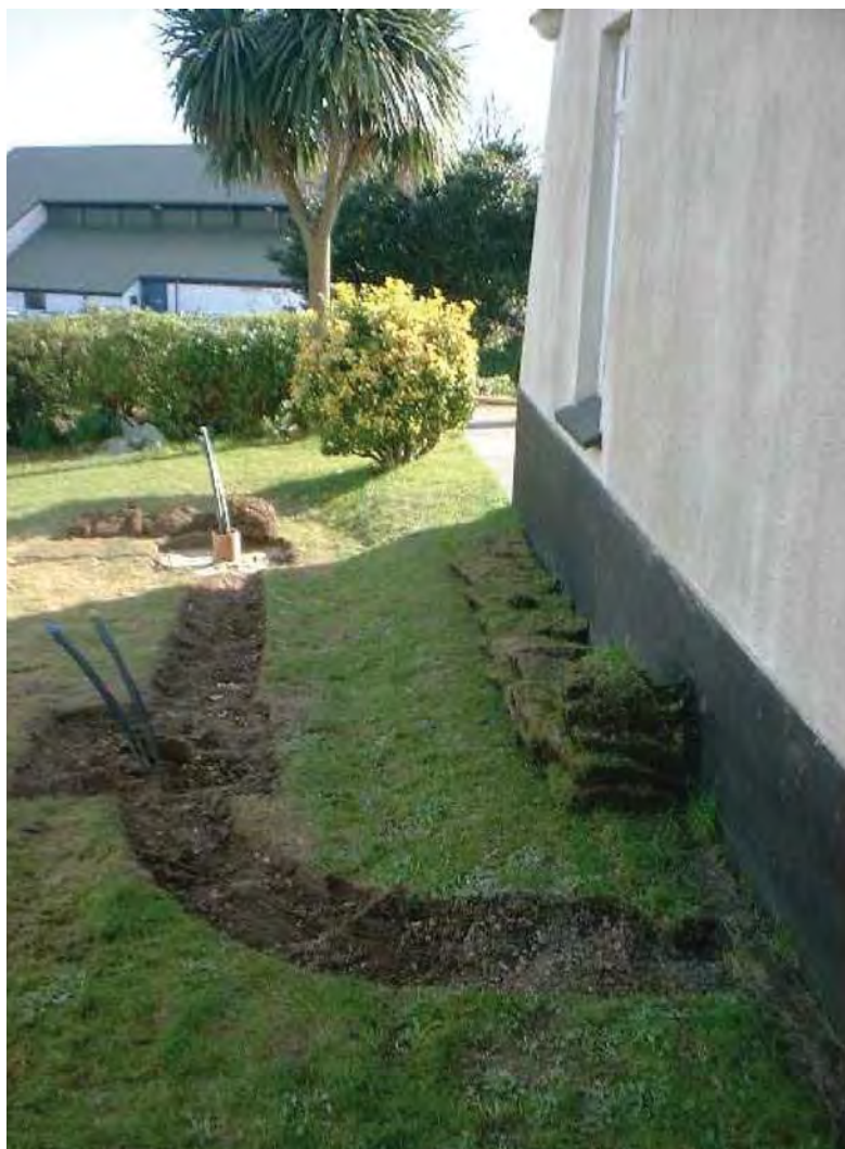
Figure 9 The heating needs of this house are supplied by a vertical collector GSHP system © Robin Curtis
