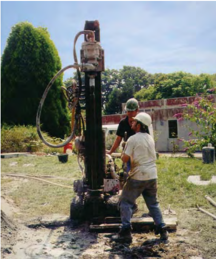
Figure 4 Typical drilling rig used for a vertical borehole based GSHP installation © R Curtis
