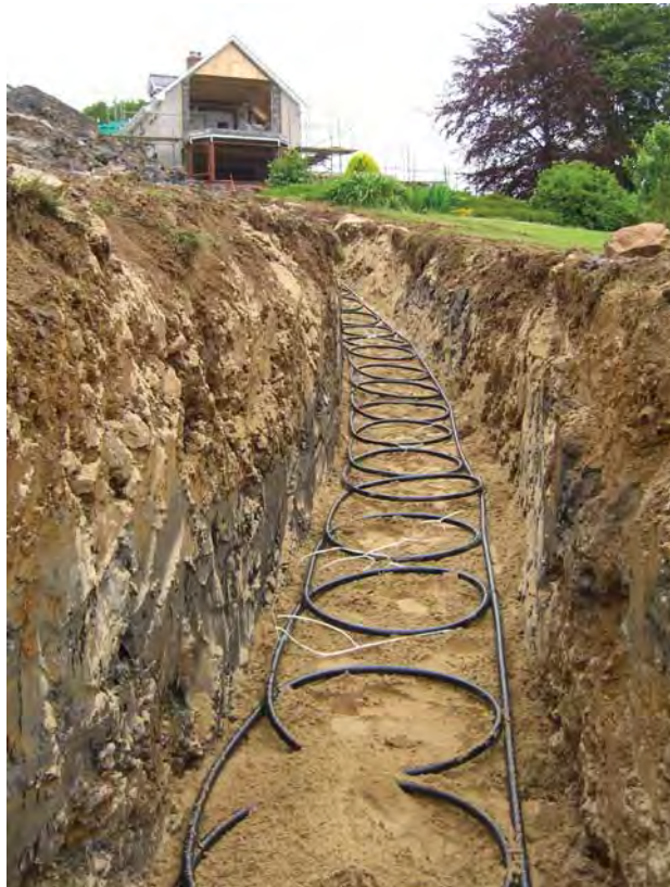
Figure 3 Trench and SLINKY™ © GeoScience
