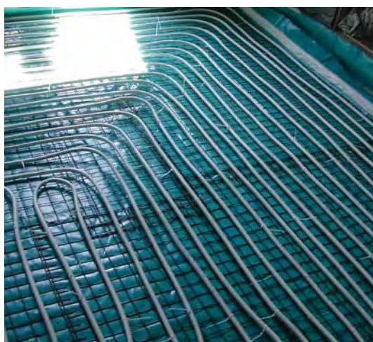
Figure 8 Underfloor heating system © J. Cantor
