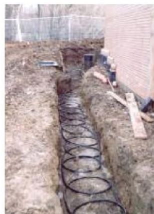
A 'slinky' ground loop being installed
