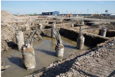
Energy Pile Installation
