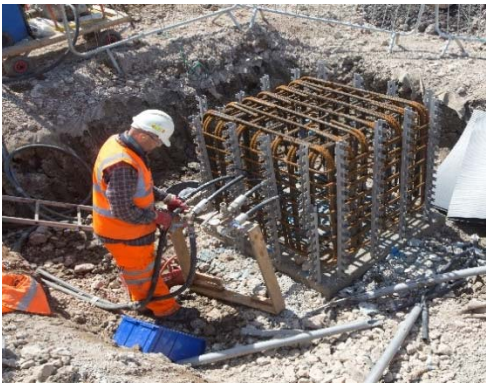
Energy Pile Installation
