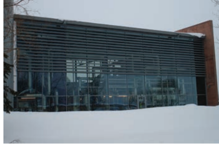
Drammen (reproduced courtesy of Star Refrigeration)
