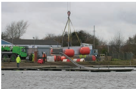
Hydroplates being installed at Kings Mill Hospital, Mansfield (reproduced courtesy of Geothermal International)
